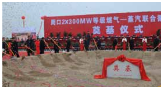
2X300MW Gas-steam circular power plant supported by Henan Branch
