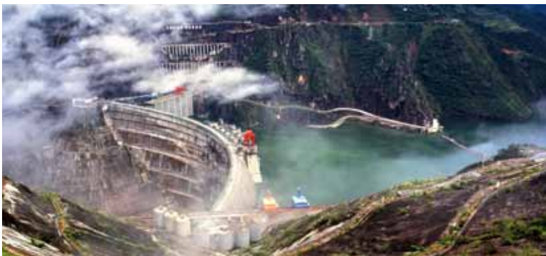
Dam of the Xiaowan Hydropower Station supported by ICBC Leasing, a subsidiary of the Bank
