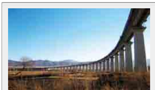
吉林分行支持的东边道铁路建设项目 The northeast railway construction project supported by Jilin Branch
